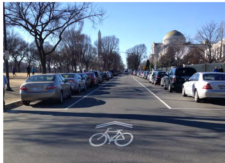
Sharrow placed in center of lane
