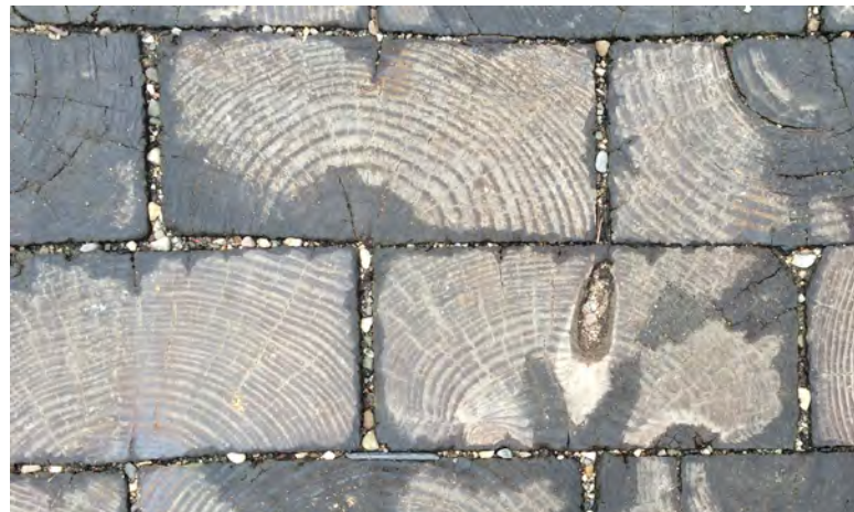
Permeable Pavers on Hessler Court
