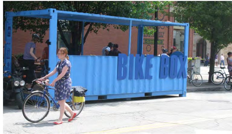
Bike Box provides low cost sheltered bicycle parking by reusing shipping containers
