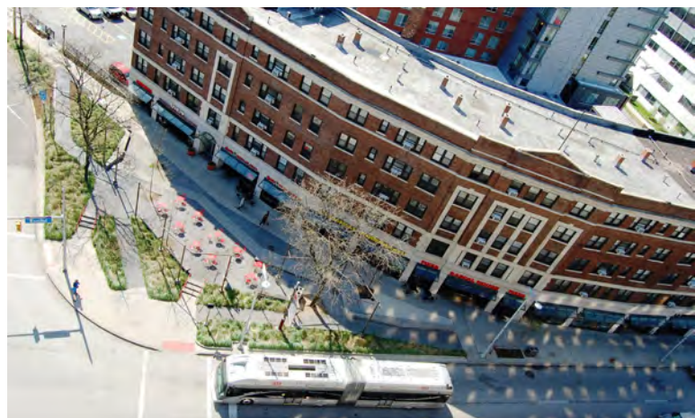
Euclid Avenue & Mayfield Road Plaza
