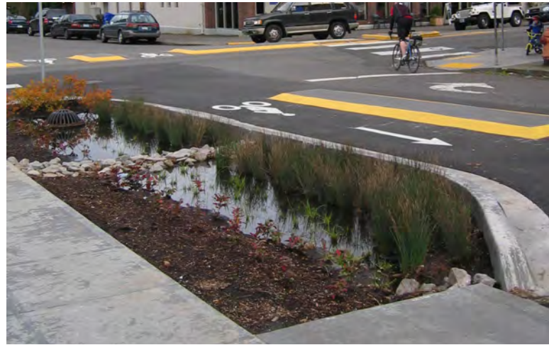
Bioswales within curb extensions create sustainable streets
